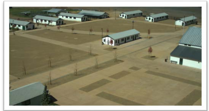
Aerial view showing concrete and decomposed granite sections.
